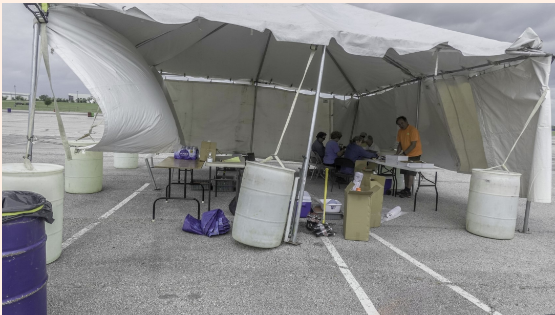
This the first hospitality tent set up for NTXCLC at Pate Swap Meet April 23rd. It failed to survive the weekend due to the Texas April winds.
